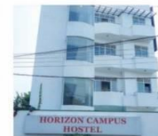
HORIZON CAMPUS HOSTEL FACILITIES
